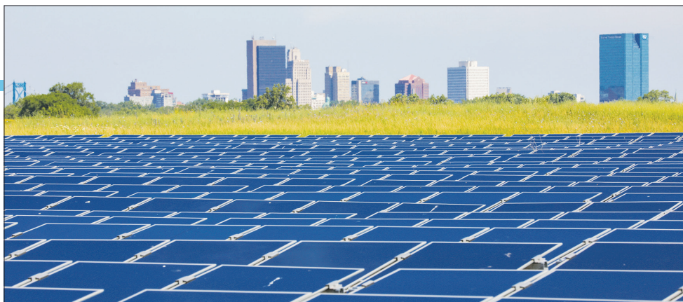
NSG Group, a global supplier of glass and glazing systems, sources solar energy for its manufacturing plant in northwest Ohio through an on-site solar field.
